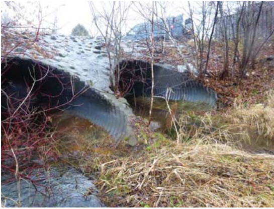
Plate 5: Culverts under Kenwood St for unnamed watercourse (November 26, 2015).
