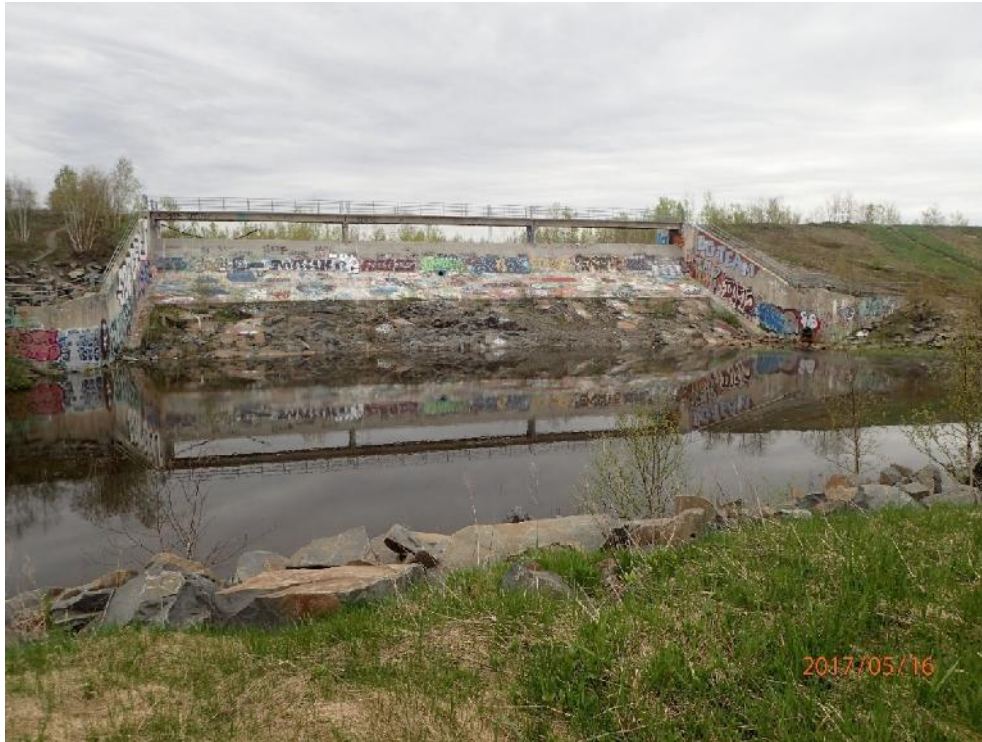
Figure 6.5.2: Photo of Nickeldale Dam
