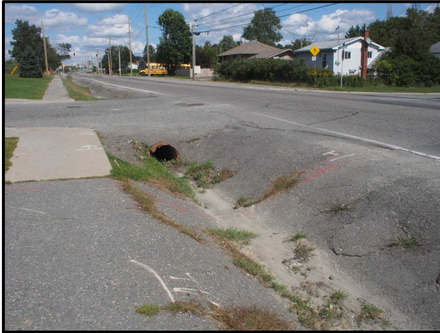
Image 9. Photograph 542 showing the sidewalk, paved shoulder, and drainage ditch on the west side of Second Avenue.
