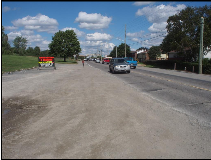
Image 13. Photograph 525 showing the disturbed gravel shoulder of Second Avenue.
