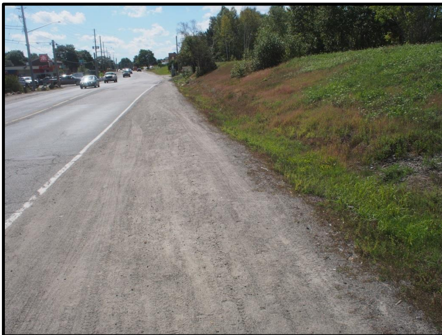
Image 6. Photograph 487 showing the gravel shoulder and a disturbed drainage feature.
