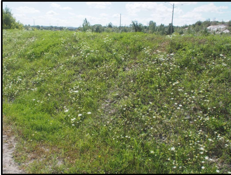
Image 3. Photograph 470 showing a raised mound on the west side of the road, a disturbance caused during the construction of the road.
