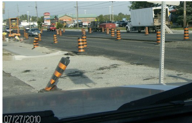
Inferior Asphalt Removed Next Day
