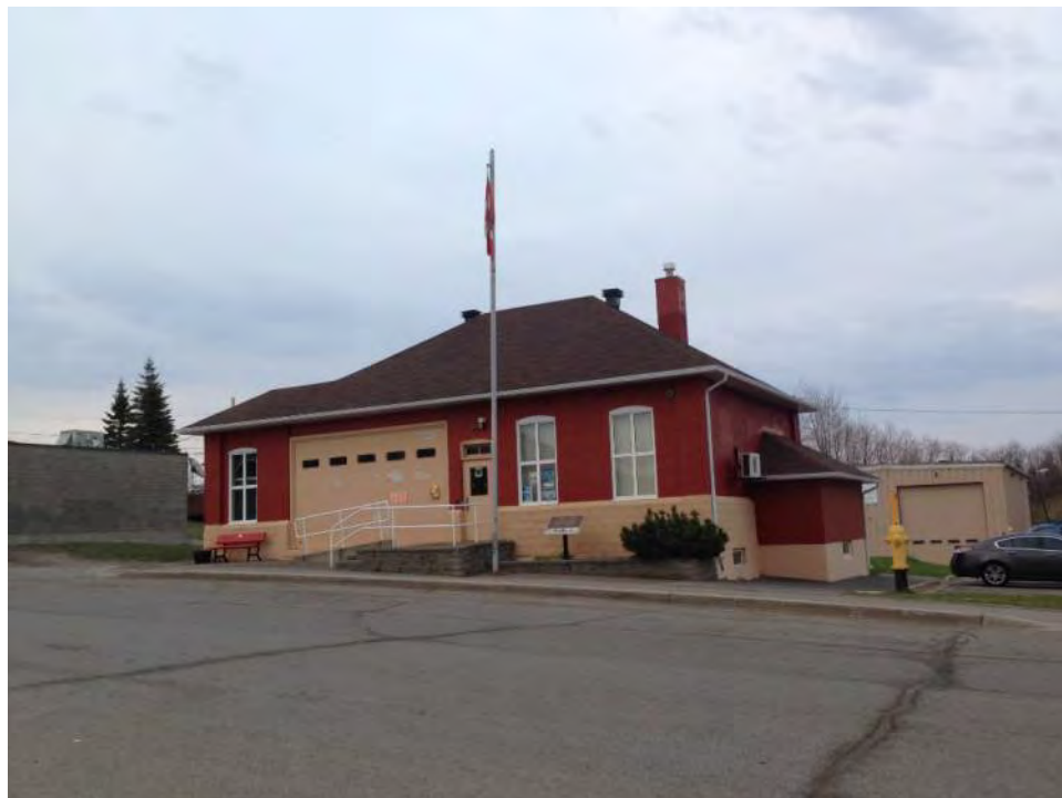
Figure 2: General view of northwest elevation.
