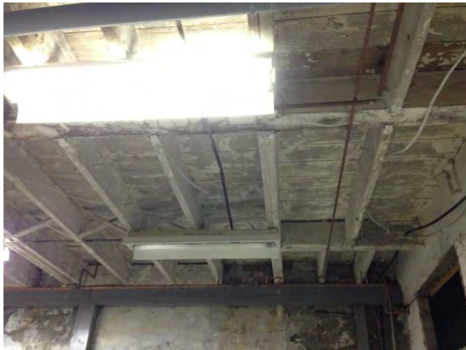
Figure 8: Original wood floor framing below concrete slab.
