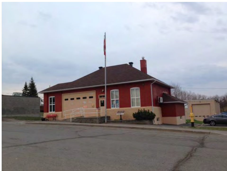
Figure 2: General view of northwest elevation.
