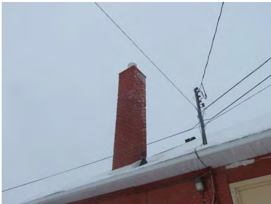
Figure 6: Brick chimney at southwest corner of roof.
