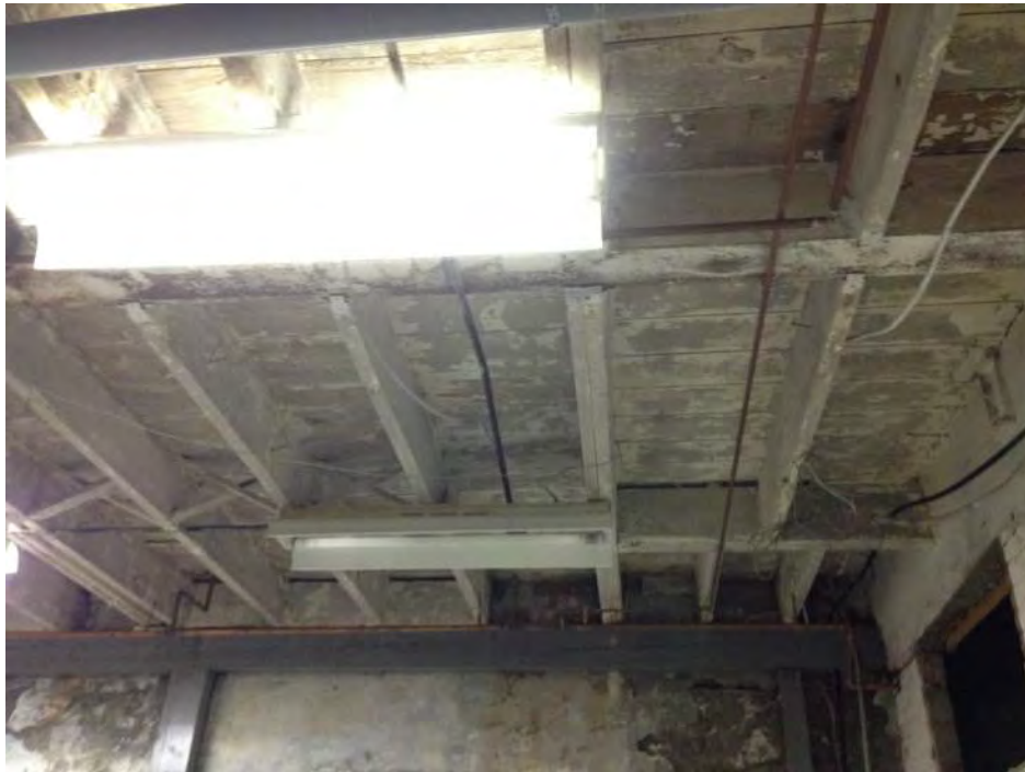
Figure 8: Original wood floor framing below concrete slab.
