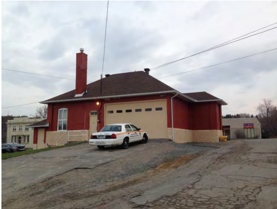
Figure 3: General view of southeast elevation.
