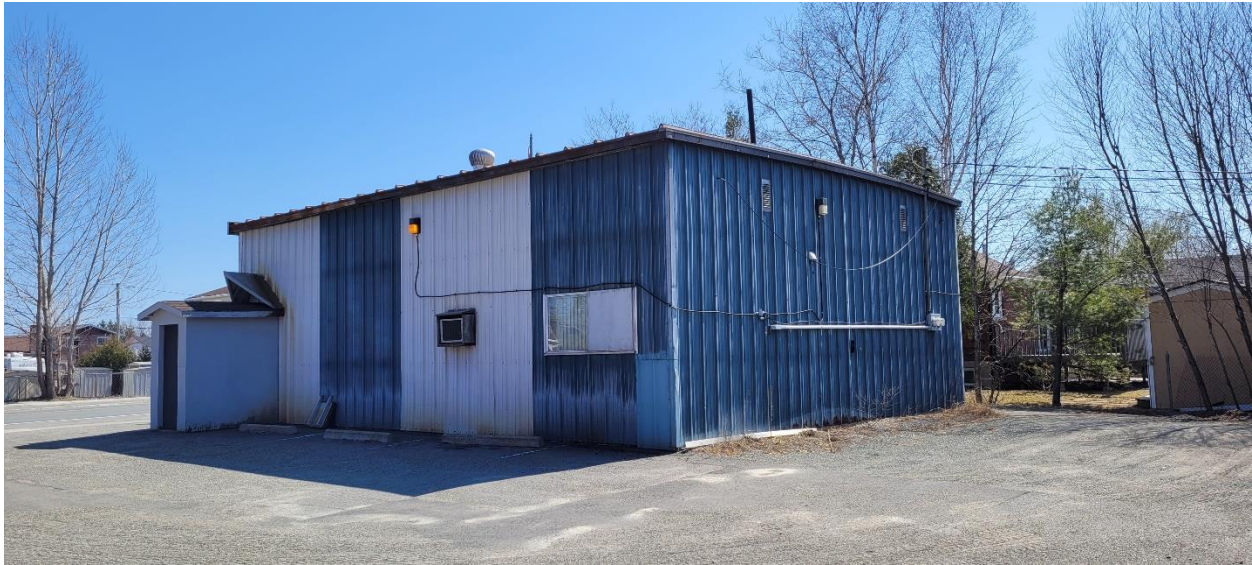
Back view of building
