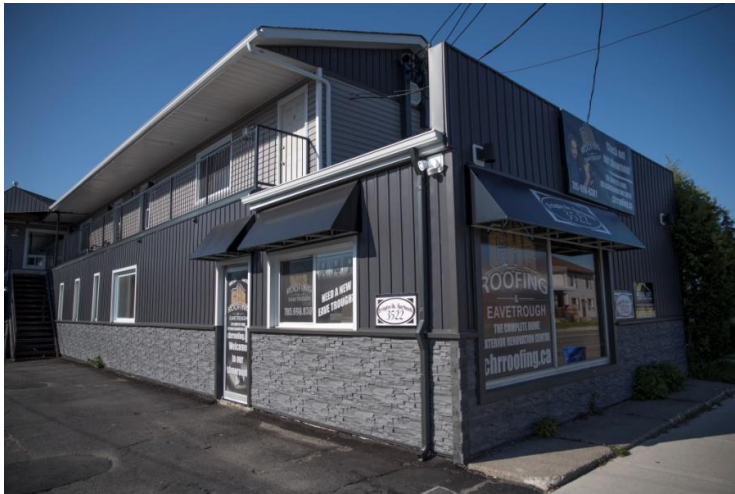
Figure 4 Redevelopment on Errington Ave. October 2017.
