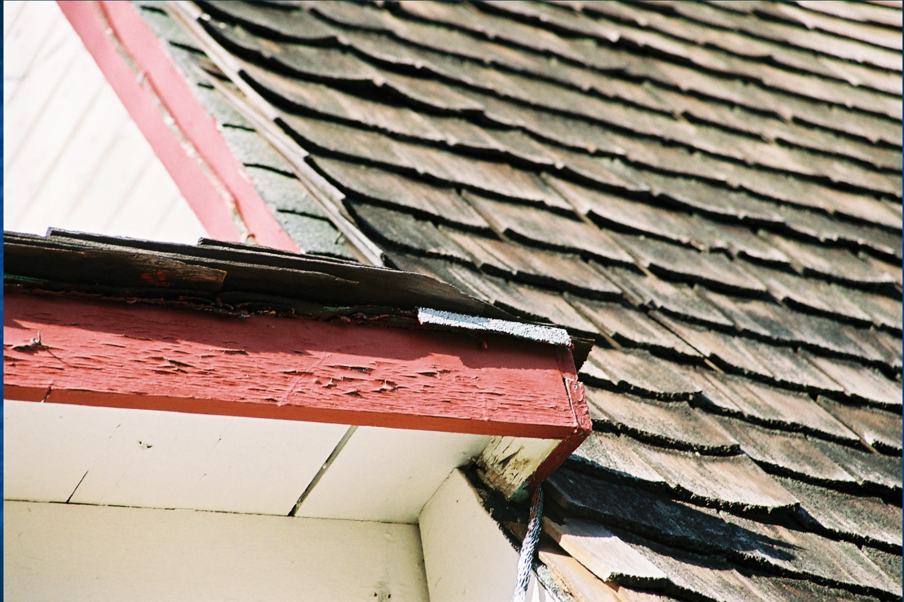
Deterioration of farmhouse roof
