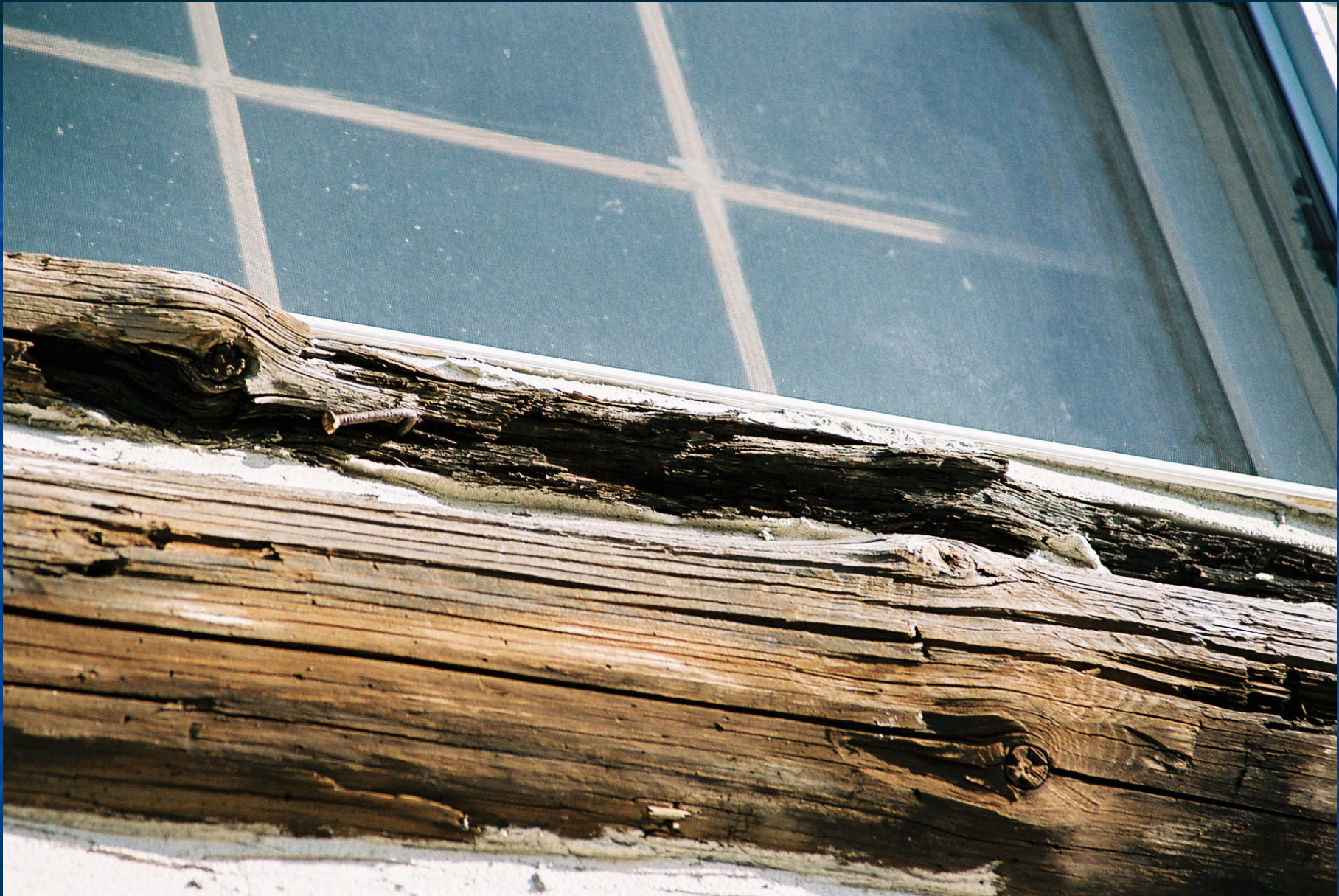
Log deterioration on Creighton building
