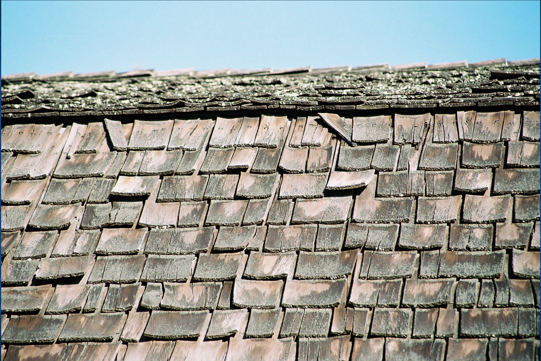
Deteriorating shingles on the granary
