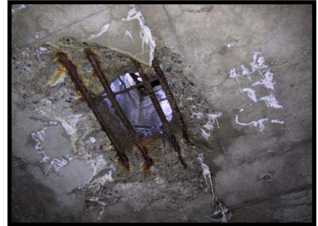
Junction Creek Box Culvert Damage
