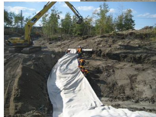
Installed GCL
