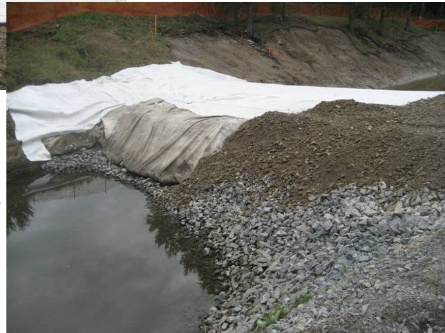
Improved Earthen Dam →
